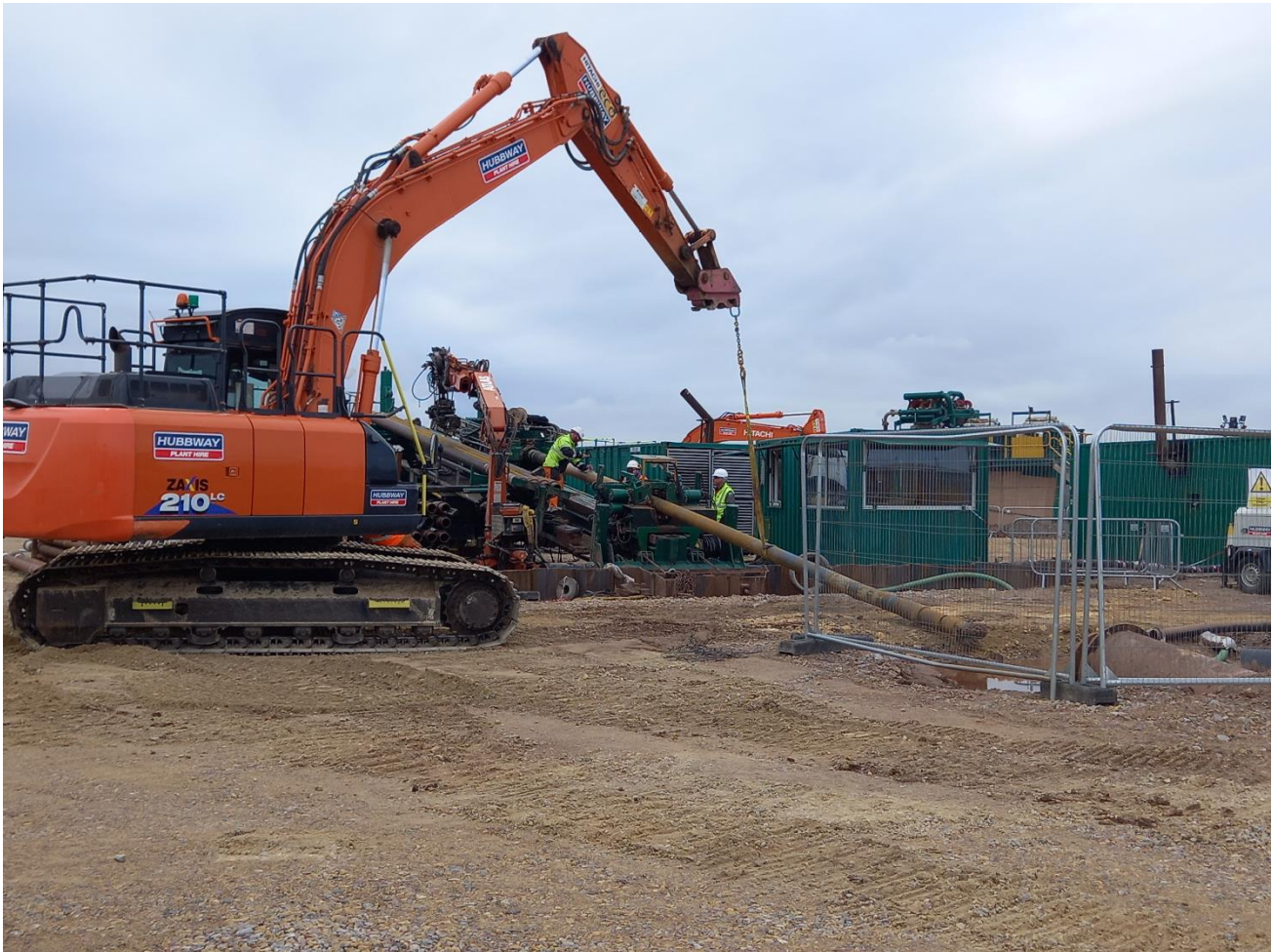
Plate 7.3 Example of Landfall HDD rig setup
