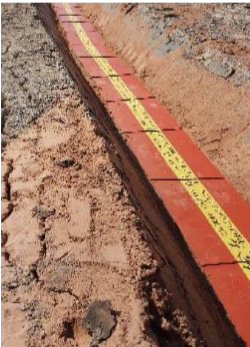
Plate 8.4 Example of protective tiles and marker tape..
