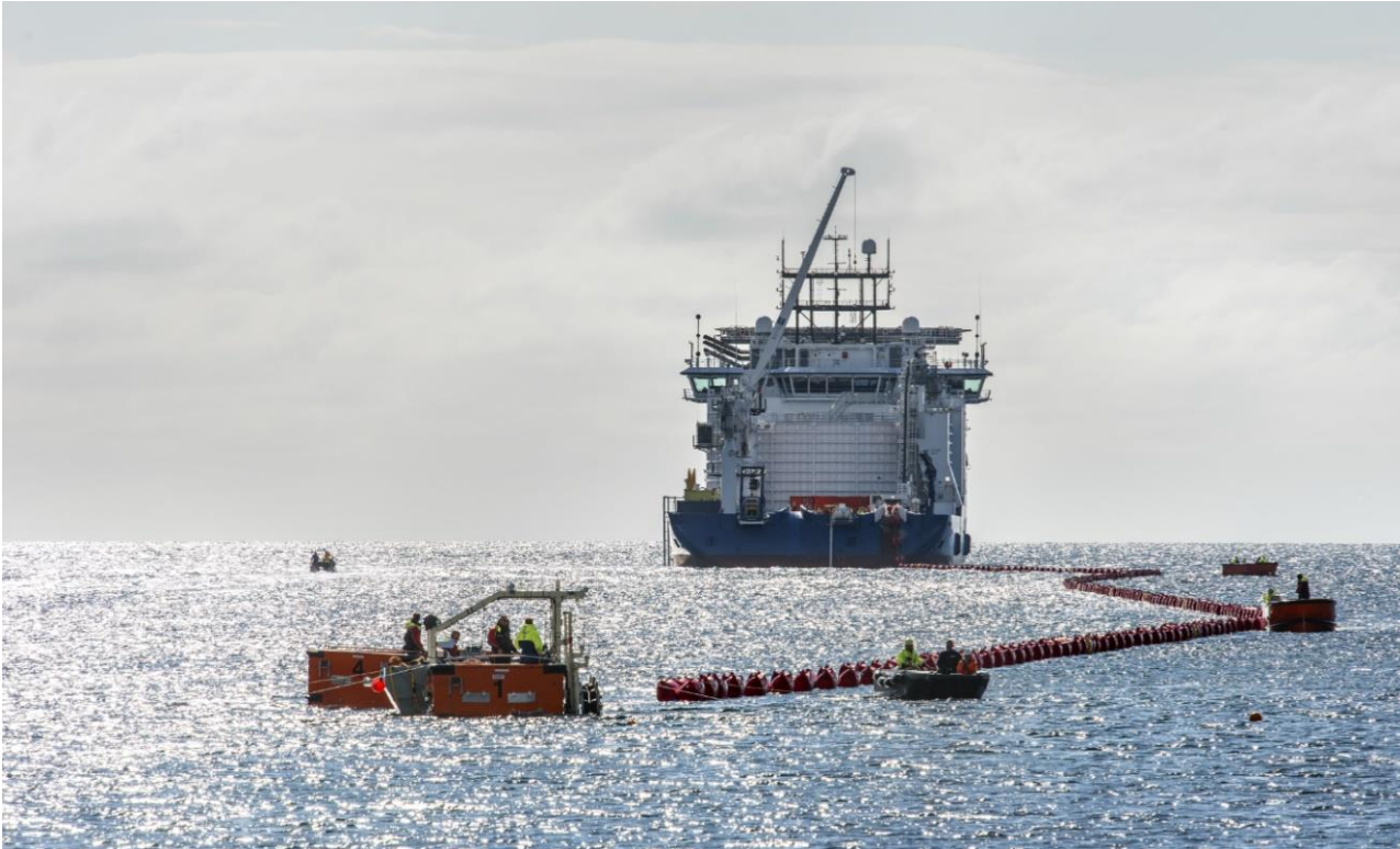
Plate 7.6 Cable pull in Source: NKT Victoria – Vattenfalls Kriegers Flak wind farm 5 .
